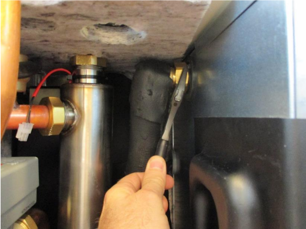
Step 17. Dismantle the upper cold carrier connection. Remove hose by pulling it downwards.
