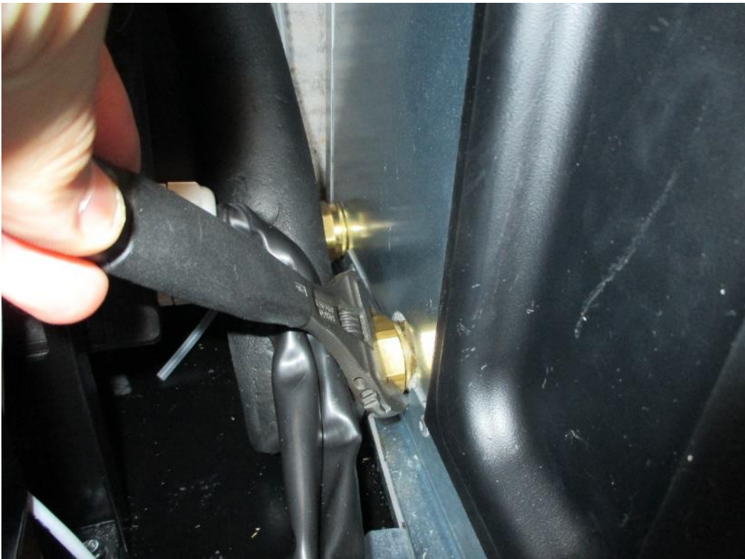
Step 18. Dismantle lower cold carrier connection.
