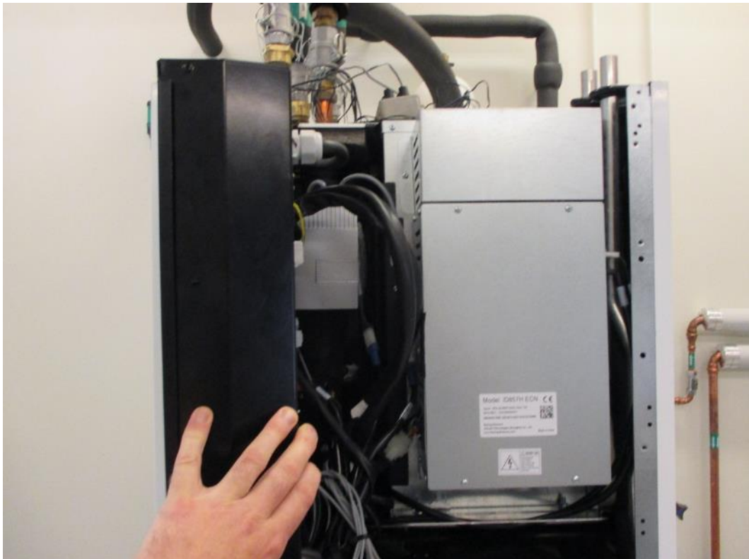
Step 6. Lift the electrical box and hang it on the left corner profile. (There is a 10 mm hole on the gable of the electrical box.)
