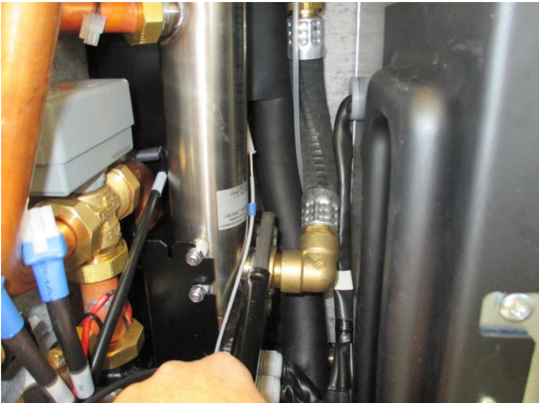
Step 20. Dismantle connection for incoming heat carrier to the electrical heater. Remove hose.
