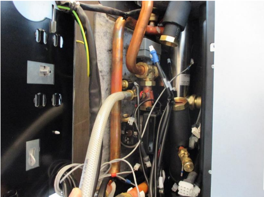
Step 16. Drain the heat carrier from the drain tap, 1/2" connection.
