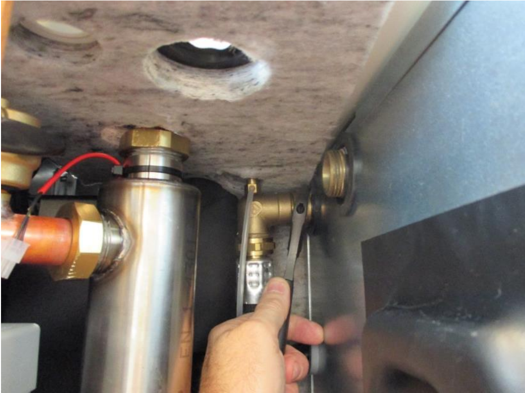
Step 19. Dismantle upper heat carrier connection.
