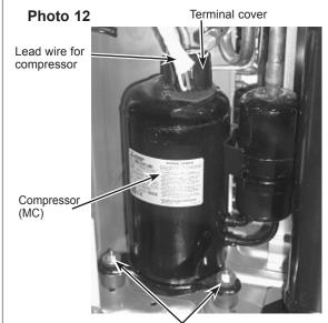
Compressor fixing nuts
