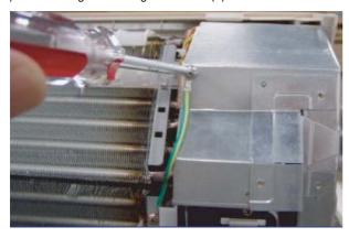
11)Remove the control box cover retaining screw (1), and remove the control box.
