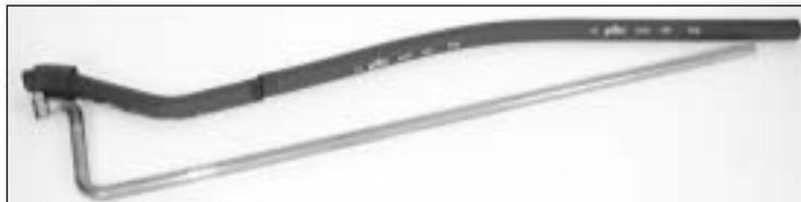
The Armaflex insulation is removed from both pipes when removing the heat transfer fluid pipe from the heat pump.
