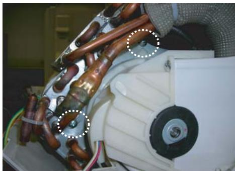
58)One screw for the drain pan fixation (right side) is removed.
