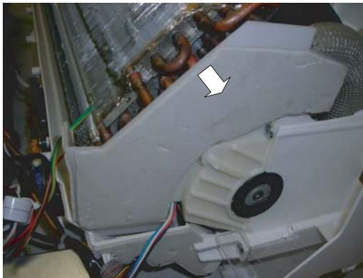
56)Two screws of cover L are removed.
