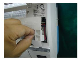
4) Remove the unit-to-unit wiring from the terminal board(4).
