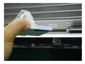
28)Remove the screw fixing the drain pan ass'y and evaporator.
