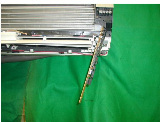
20) Disconnect the connector of Display board.
